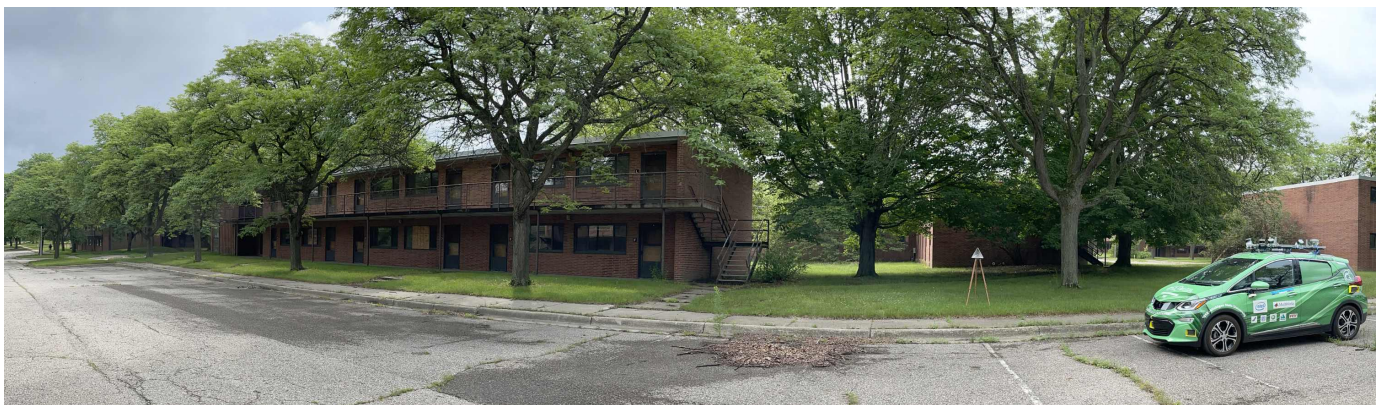
Fig. 15. Ground-based optical image of SAR track three. The corner reflector is shown near the right side of the image. Small steps can be seen in the sidewalk leading up to the building between the trees on the left side of the image.
