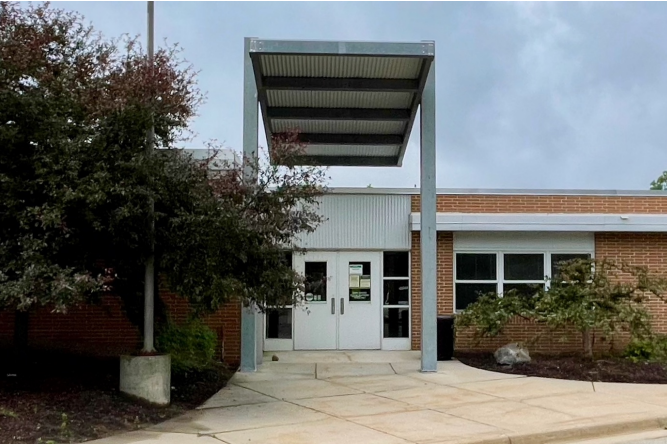
Fig. 9. Ground-based image of the awning highlighted in ROI 2 of Fig. 6.
